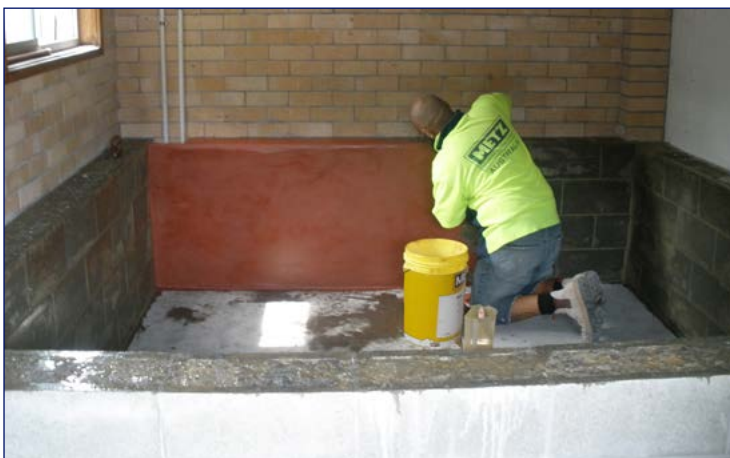
Chemical storage areas require a lining that will resist concentrated chlorine and acid. Metz manufactures a range of materials suitable for all such areas.
