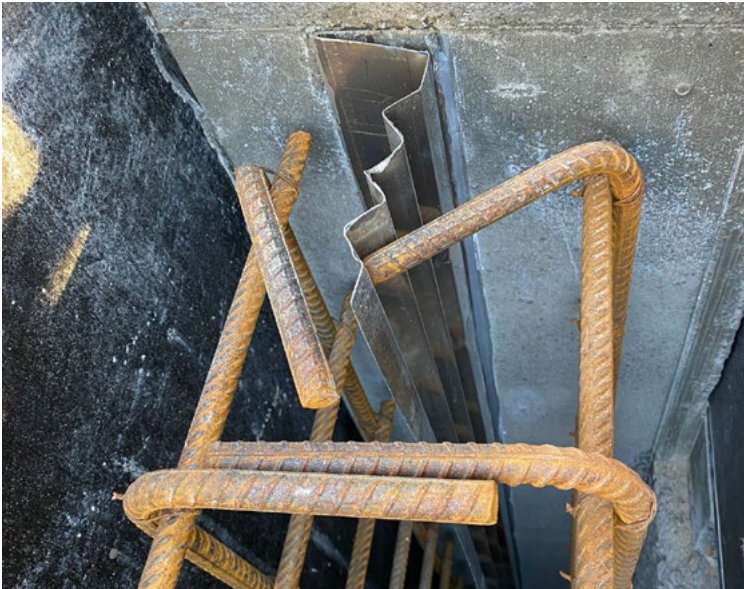
Rebuilt well using acid resistant concrete and stainless steel waterstop
