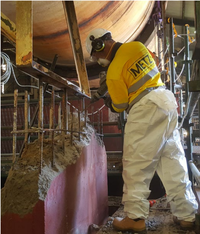
Remediation during shutdown of a concrete column corroded by chemical agents
