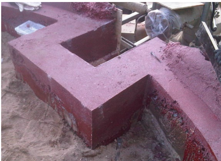
Repairs to a chemical tank base
