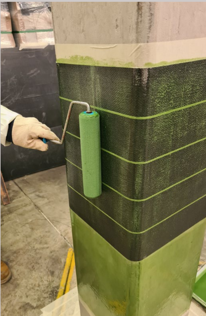
Carbon reinforcement to increase the strength of structural elements
