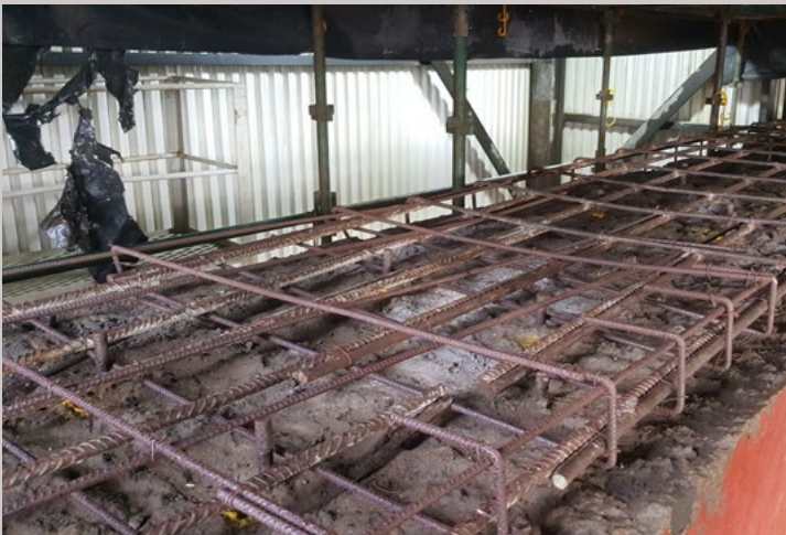
Rebuilt support beam coated with Metz Epoxy material after demolition
