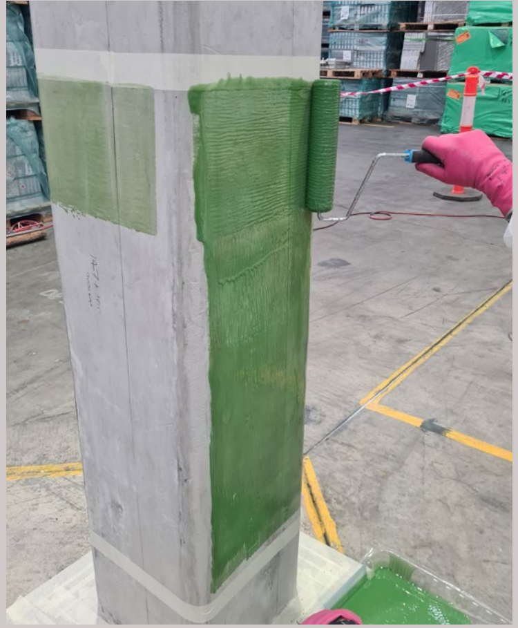
Application of the self priming impregnating resin Metz C100
